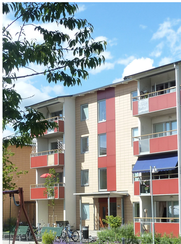
Buildings after refurbishment
