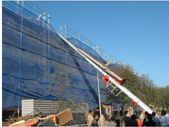
Roof elements assembly
