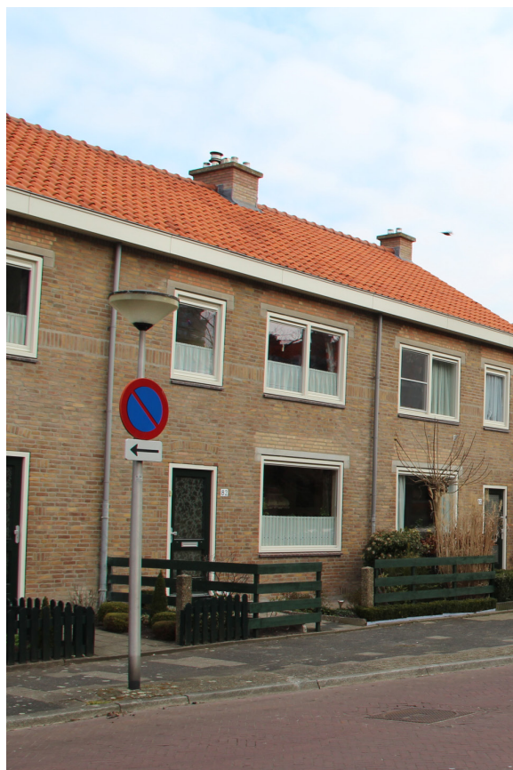
The building after refurbishment
