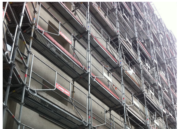
Construction work on the back facade of the building
