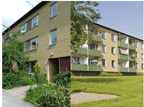
Building before refurbishment
