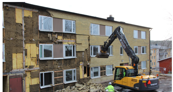
Demolition work at Brogården; the original façade is taken down
