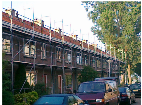
Refurbishment works in Delft pilot site
