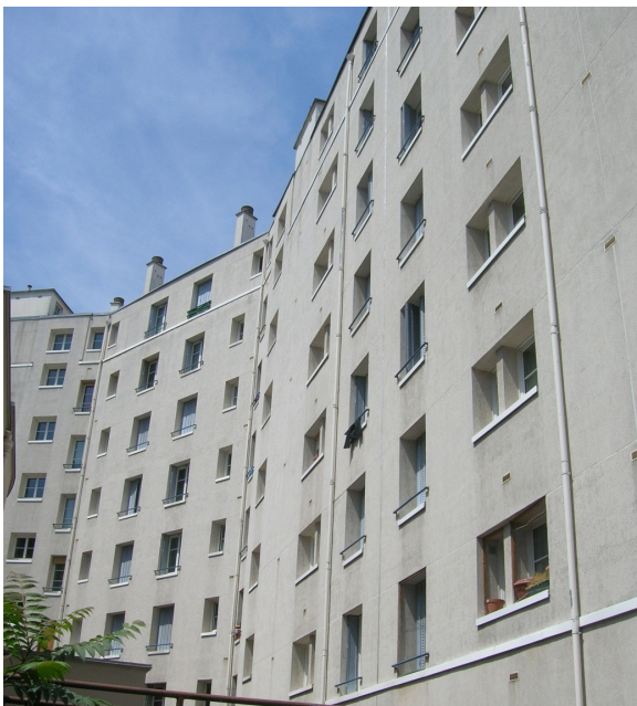
Back facade before the refurbishment
