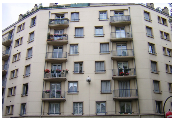
Paris building before the renovation
