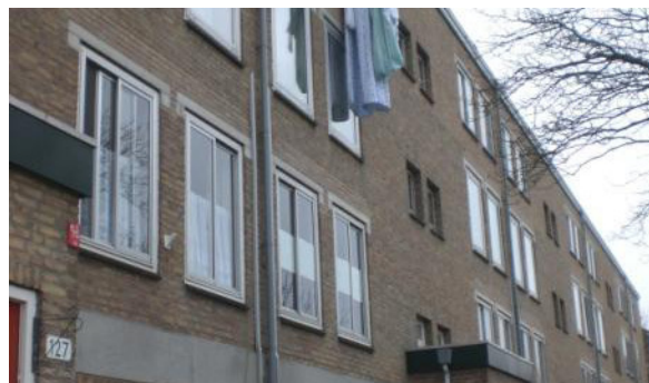
Building before refurbishment
