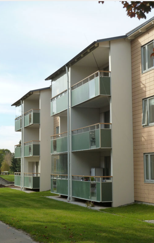
Externally mounted balconies
