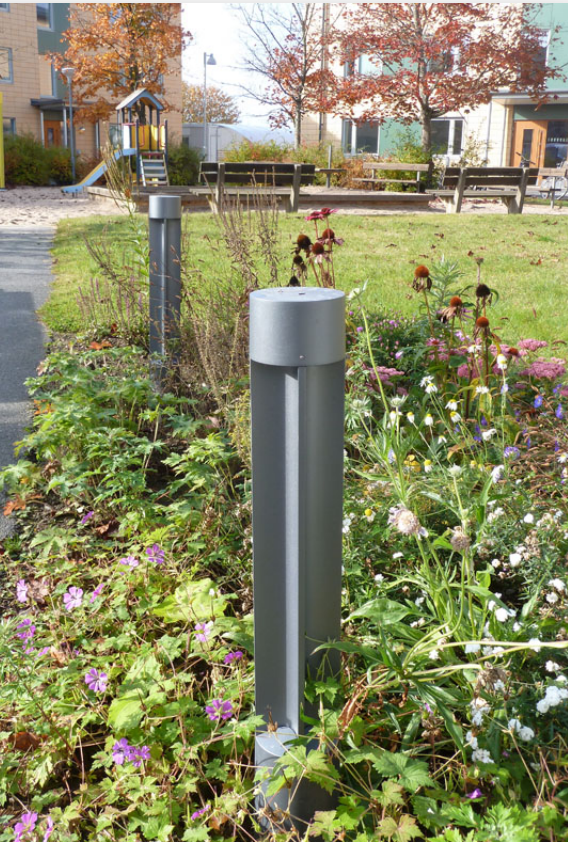
External light fittings
