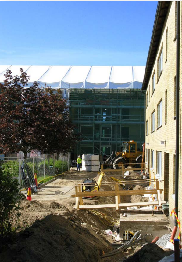
Work in progress on the foundations
