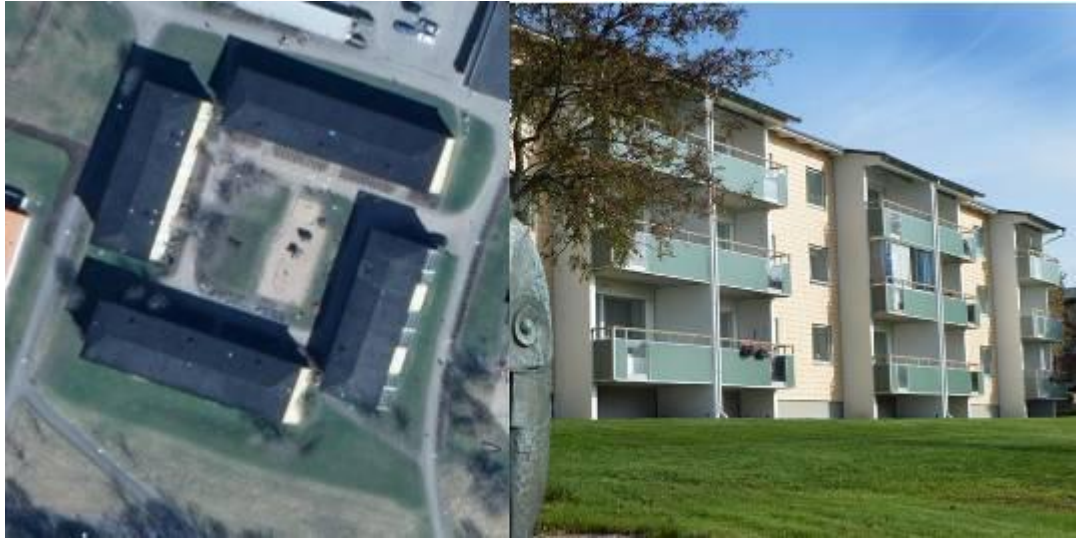
Fig. 4.3. Left: Satellite picture over houses N, O, P and Q. Right: Refurbished balconies at house E
