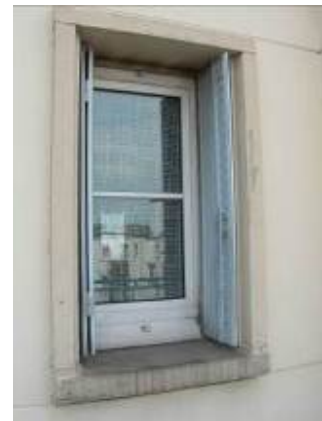
Fig. 6 PVC windows with metal blinds
