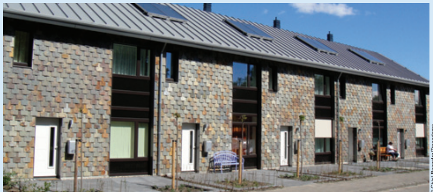
Demonstration building in Roosendaal, the Netherlands, after retrofit.
