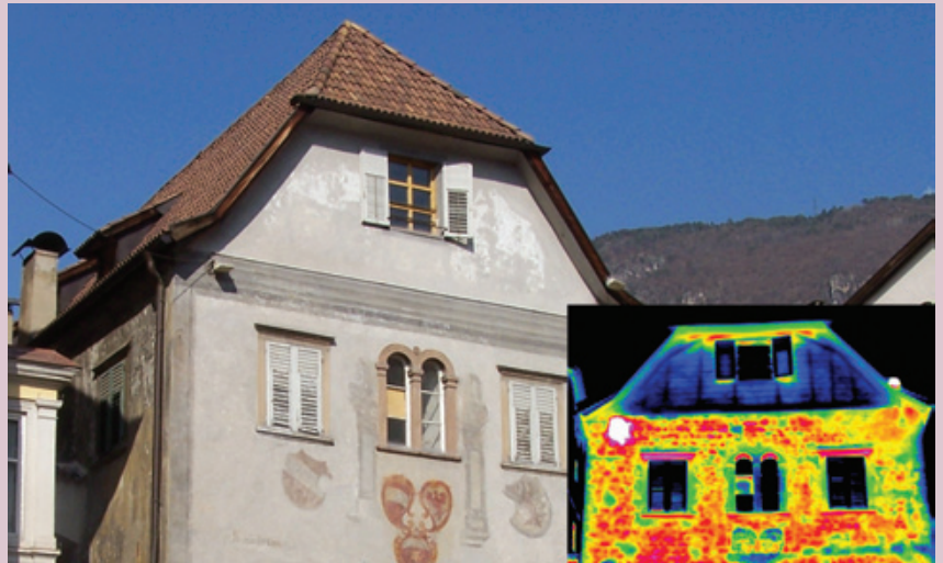
Thermography of the Public Weigh House in Bolzano/Bozen (Italy)
