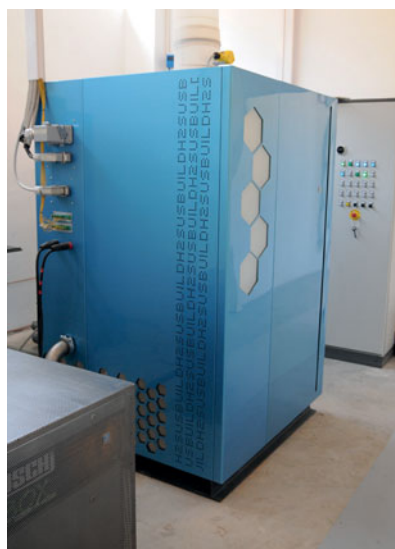
Fuel cells based 20kW micro-cogeneration system
